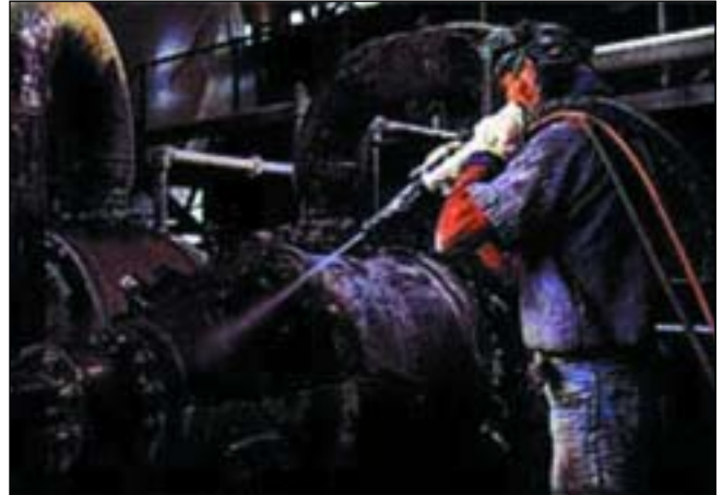
Specialised equipment is needed for sodium bicarbonate blasting.
