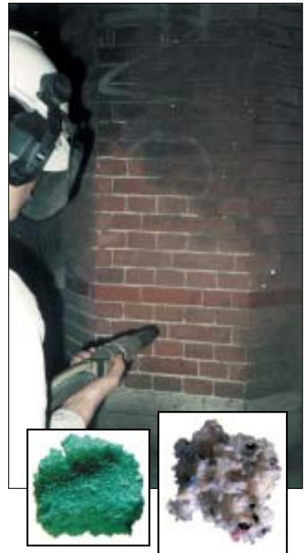
One use for sponge blasting is removing soot from brick and other substances. Courtesy of Sponge-Jet, Inc.
