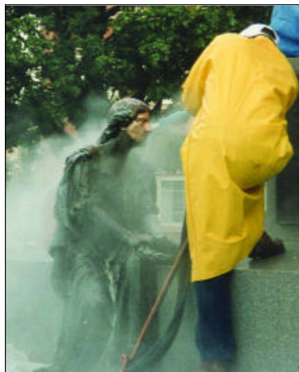
Using sodium bicarbonate for restoration work. Courtesy of Armex®
